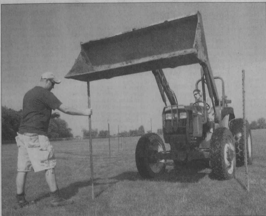
Pat Davison uses the bucket of the tractor to drive in a stake held by Joel Judycki. They are building a fence for the Canton Cup soccer tournament.
