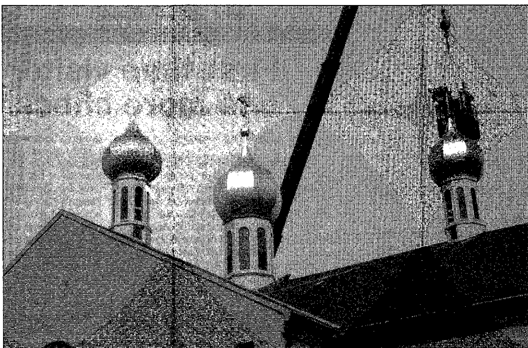
A crane raises one of four new cupolas to the roof of St. Michael the Archangel Russian Orthodox Church in Redford.
