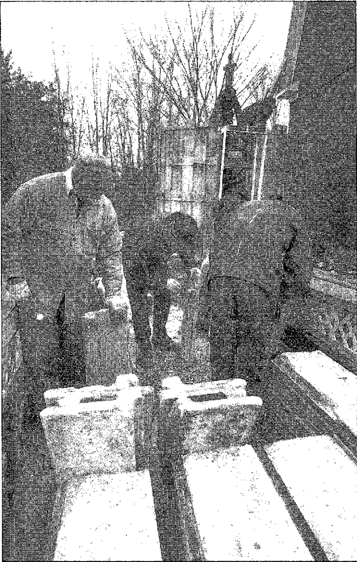
The cast concrete plates weigh 60 pounds. They are cleaned so they'll fit together easier, hoisted up to the work platform and then are hand-fit in place.
