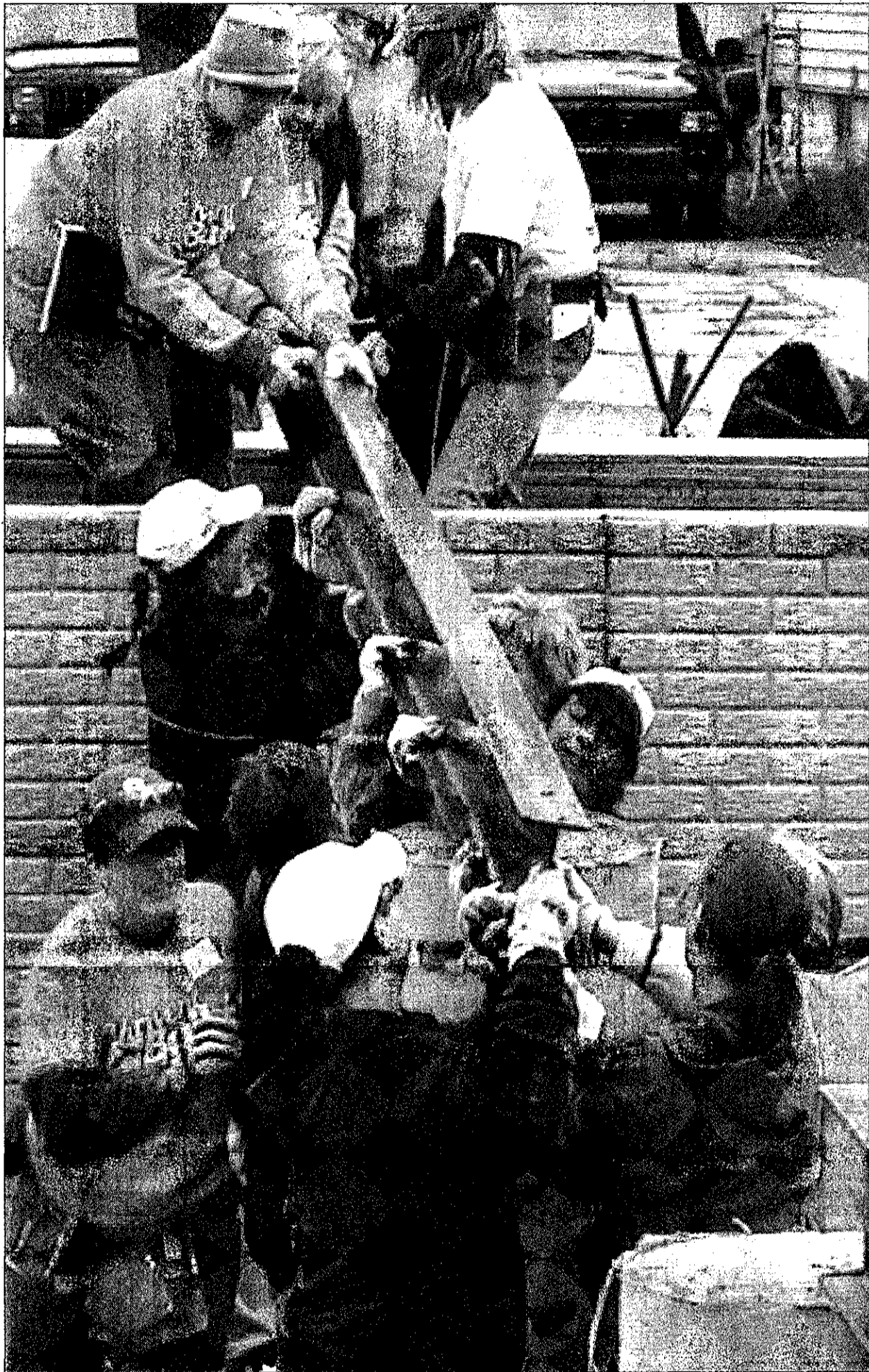
Girders go in place during the recent Women Build event in Pontiac. Some 25 women volunteered at the construction site for Habitat for Humanity of Oakland County. The build was also sponsored by Thrivent for Lutherans.
