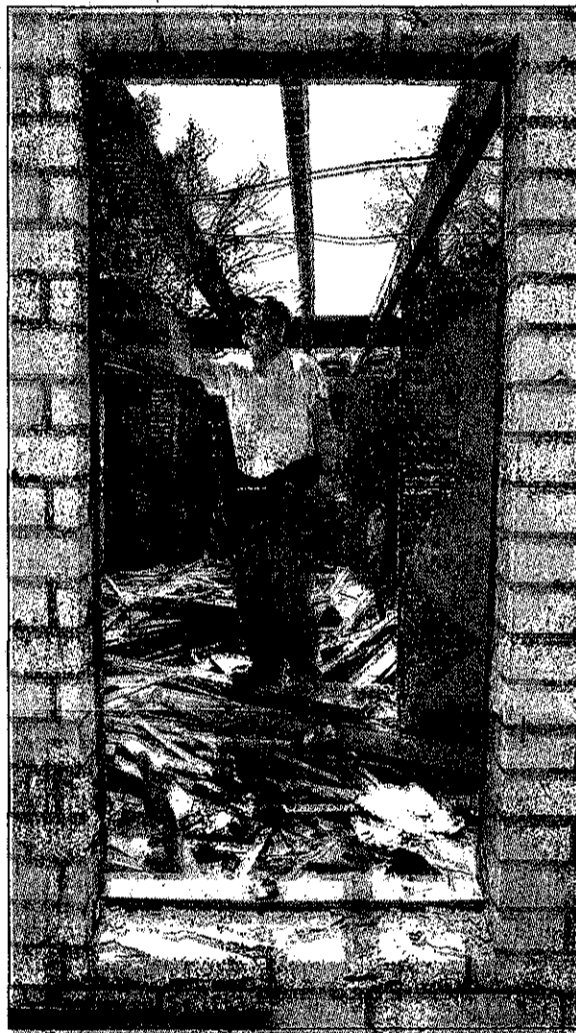
The original frame of the building will be saved. Robert Babbitt works on the deconstruction.
