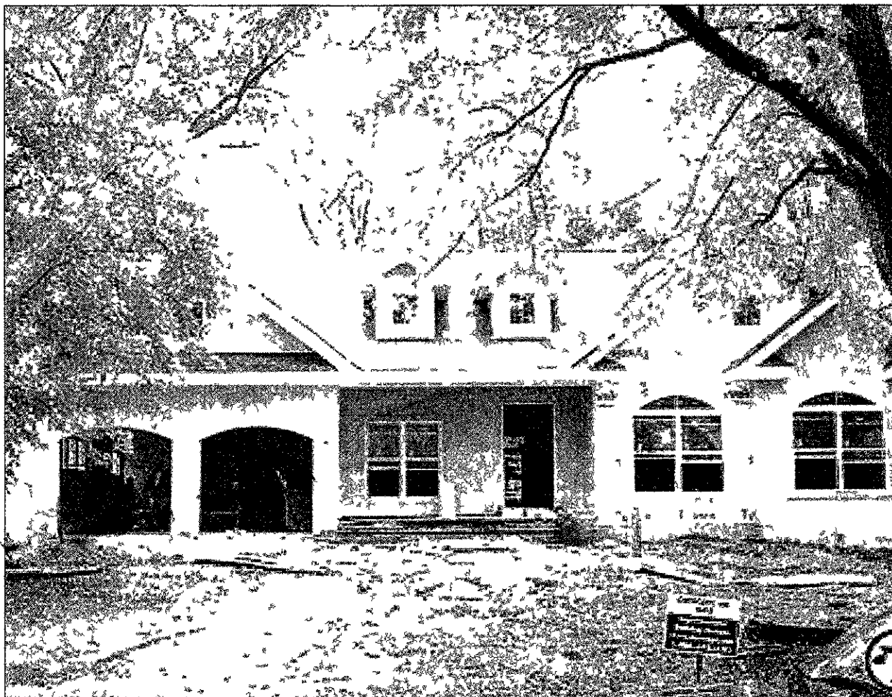
This green home is being constructed using energy efficient and environmentally friendly building techniques.
