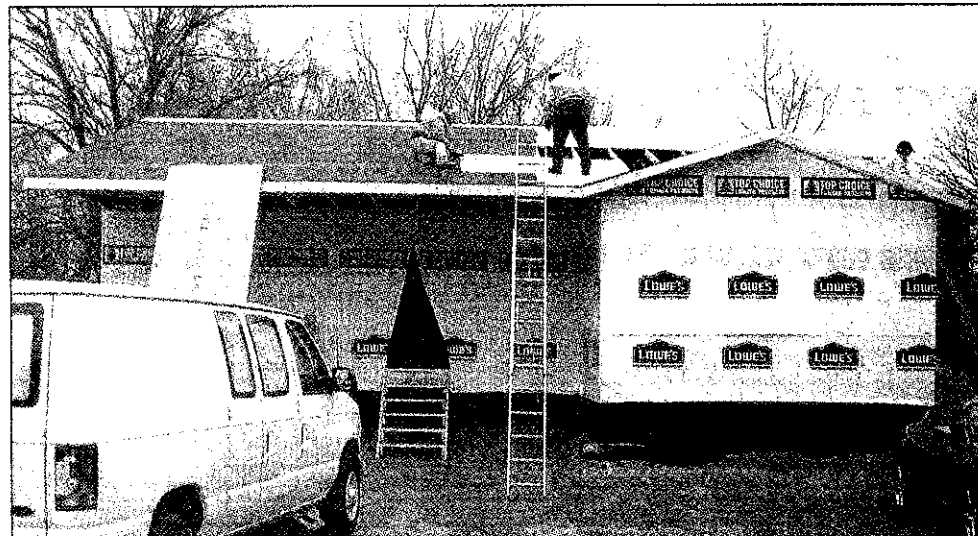
Workers construct the Belleville home's roof.
