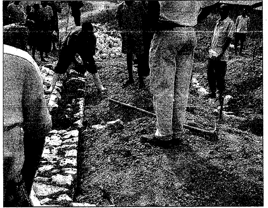
Building a mud brick house for a widow in Rwanda was part of the work for the Food for the Hungry mission group.
