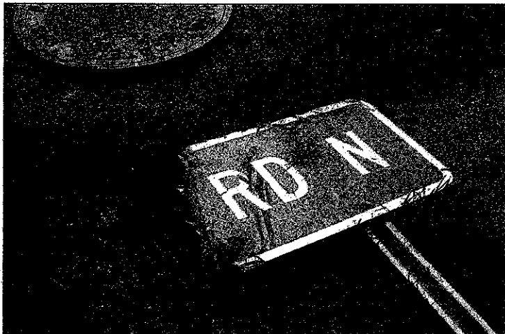
Construction along and on Cherry Hill Road continues.
