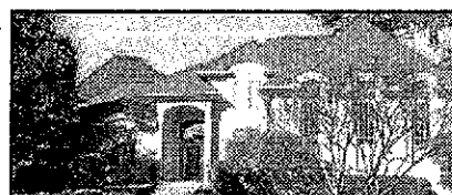
ROCHESTER HILLS Transferred Executive Private cul-de-sac location. First floor master suite with fireplace, walk-in closet, 3 bedrooms, 2 baths up, kitchen with island, great room fireplace, sun room off nook, partially finished lower level with cedar closet. (B37CRO) 248-652-8000 $574,000
