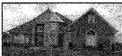
WASHINGTON Orchard Golf Course Magnificent custom home w/cathedral ceiling in GR, beautiful fpic and stunning spiral granite staircase. Porcelain flrs w/granite trim, 1st flr mstr suite, gourmet kit w/granite counters, 4 BR's and 4 car garage. (B41PIN) 248-652-8000 $715,000
