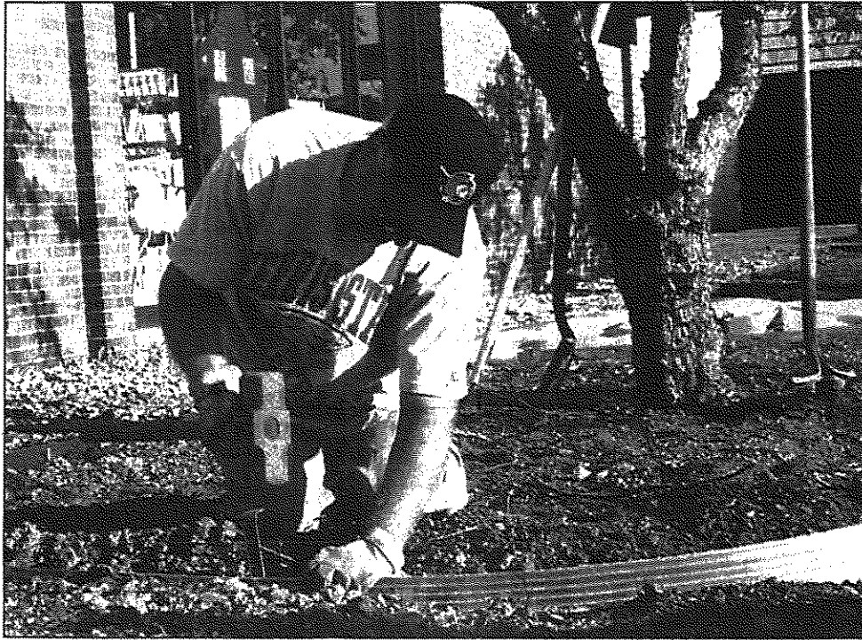
New aluminum edging is shaped and hammered into place by Fred Bizovi. This edging will provide a clean barrier between the plant material area and the mulched area.
