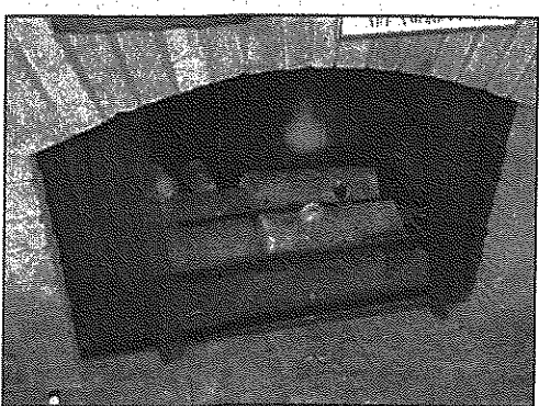
Above, adding two inches of Styrofoam insulation between joists and in the area of an old basement window can prevent heat from escaping. Below, this fireplace could use a glass door on it to prevent heat loss.
