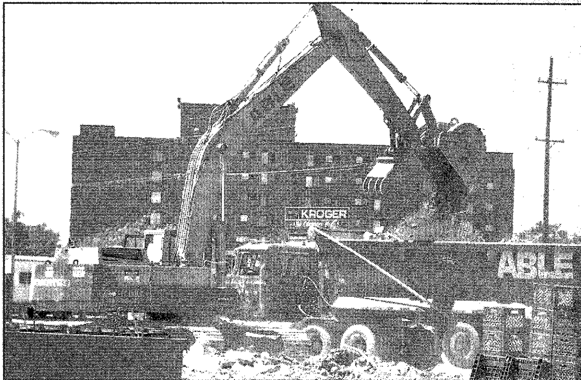
Getting ready: A demolition crew cleans up the remains of the Kroger store on Ford Road and Sheldon last week. A Walgreens drug store will be built in its place.
