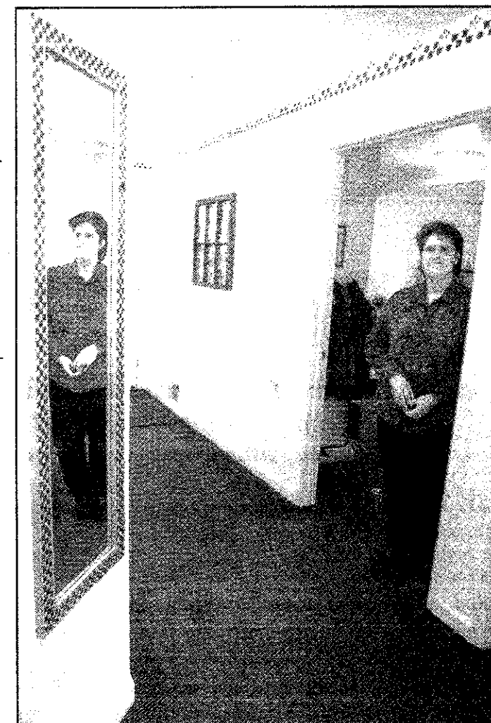
Down the hall: Kathy Renas stands in the widened doorway of daughter Lydia's room adjacent to a hallway built wider than the standard 36 inches.
