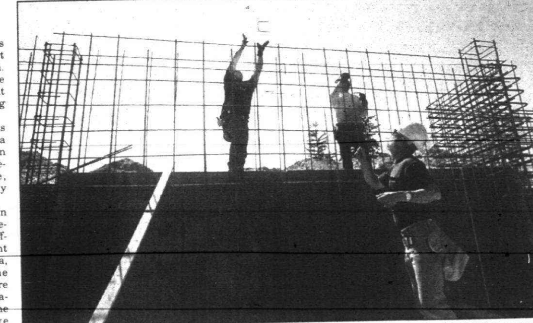
On schedule: Steel workers from Raven Resteel tie steel supports in the south wall of the new 35th District Courthouse in Plymouth.
