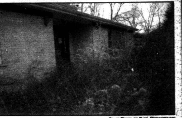
Empty: Currently, weeds and tall grass mar the facade of the property of the abandoned home.
