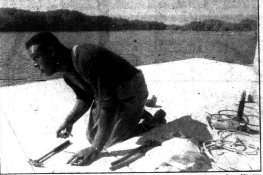
Finishing touches: Lyle Rodgers from Inland Marine in Ferndale installs a new fishing dock on Newburgh Lake.
