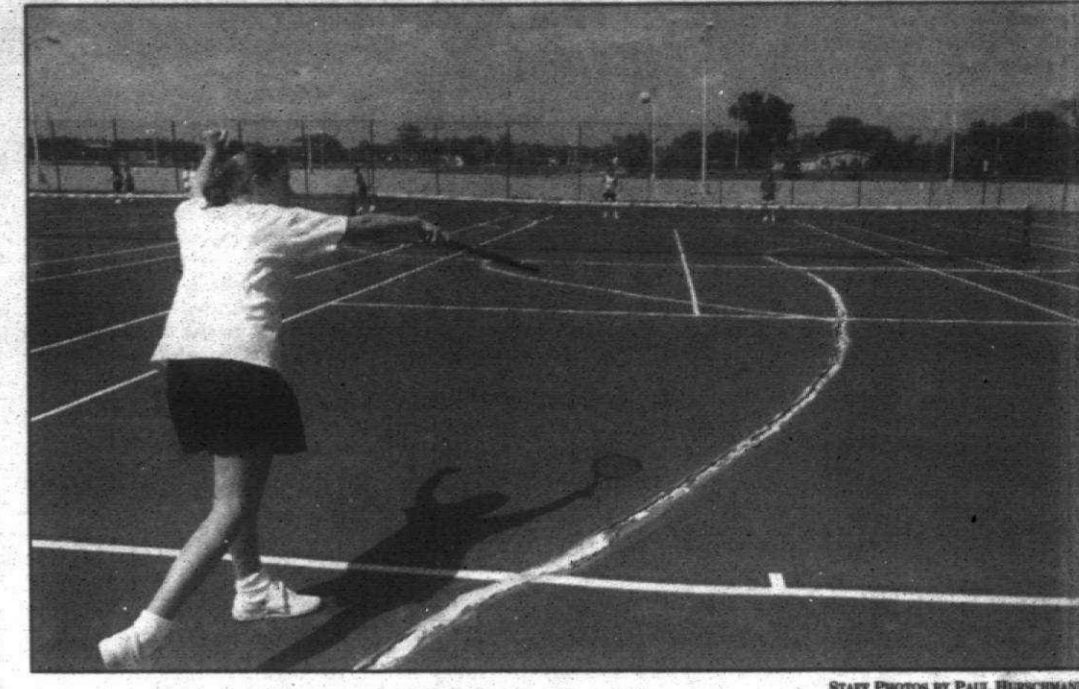
Rough shape: Melanie O'Neil practices on one of the PCEP tennis courts this month. The playing surfaces of the courts are uneven, cracked and there are large protrusions in the center of each court. Court Five is in such bad condition that coach Barbara Hanosh does not allow her players to practice on it.
