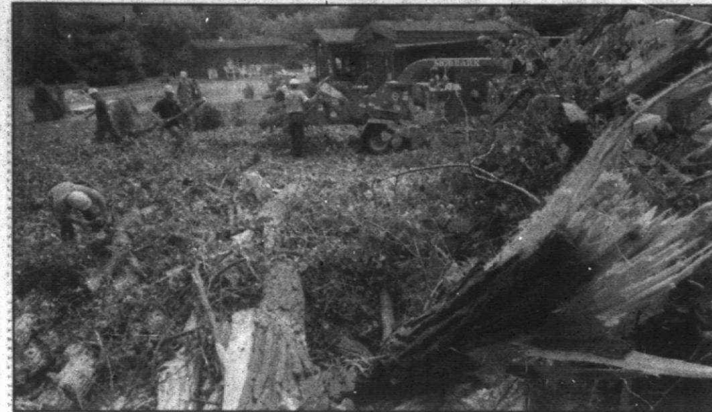
Heavy duty: Work crews clear away fallen trees and limbs from James Wood's home on South Road in Canton Friday. Wood said he lost three or four trees on his property in Tuesday's summer storm. One tree crashed into the house, breaking windows, gutters and ruining siding. Wood estimated a cleanup bill of $3,000-$4,000 and overall damage of $10,000-$15,000 to his property.
