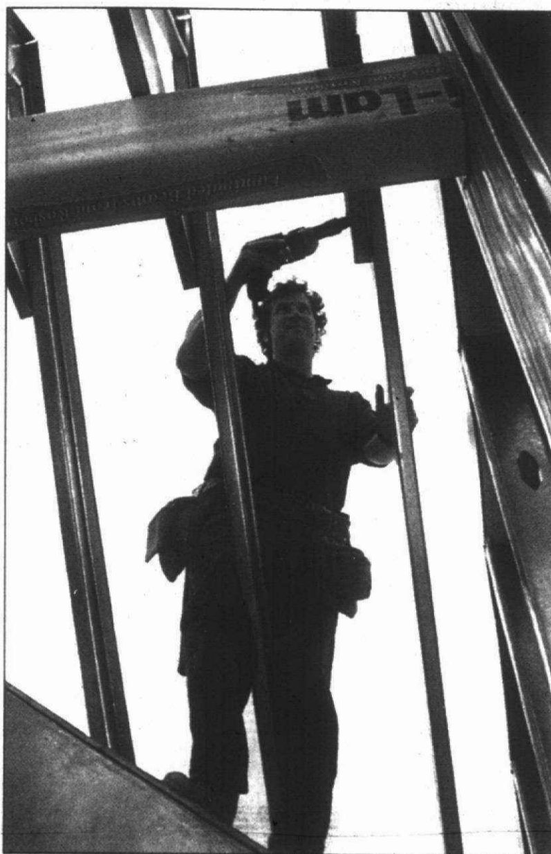
Man of steel: Dan Hall fastens steel beams with a power screwdriver. The metal-framed home he is building on the Pheasant Run Golf Course is a first for Canton.
