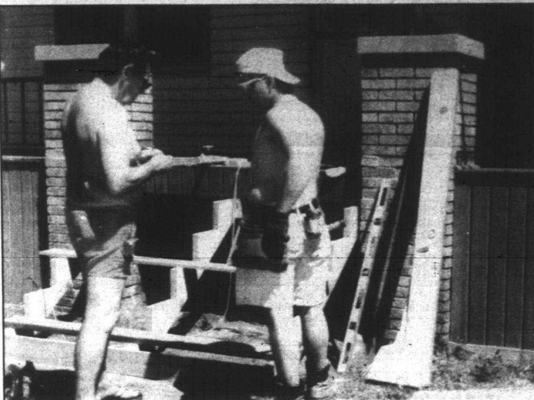
Checking it twice: Dan Rimer (left) and Mike Andridge double check their measurements while replacing the rotted front steps on Stan Michalski's home.
