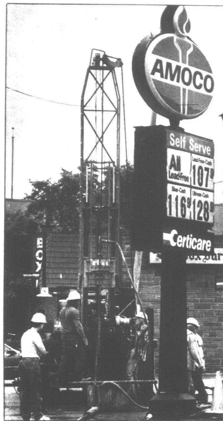
Work continued at the Amoco station on Main in Plymouth last week, as workers drilled into the ground to measure how far contamination from oil leaks had spread.
