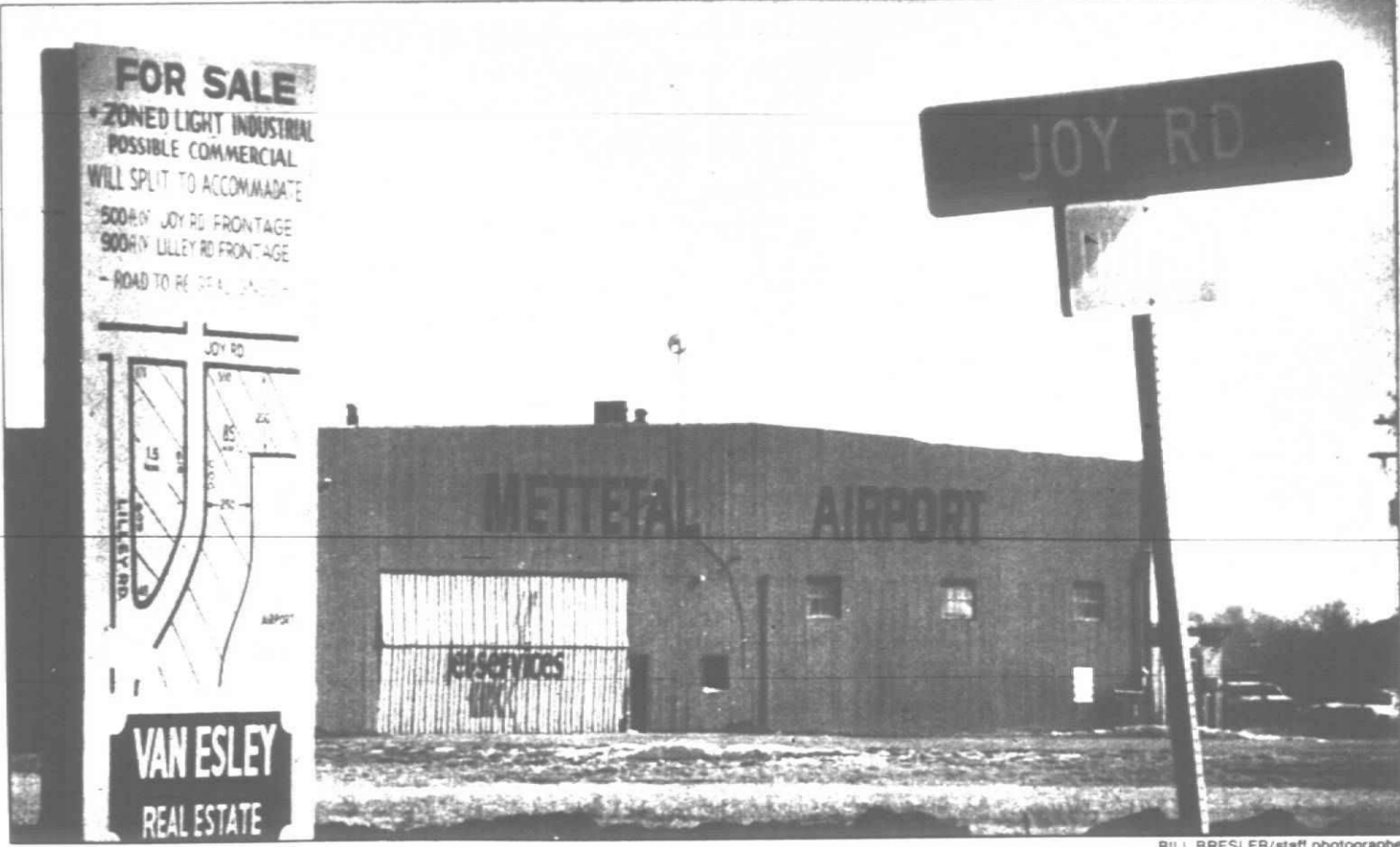
Work is under way to realign the intersection of Lilley and Joy.
