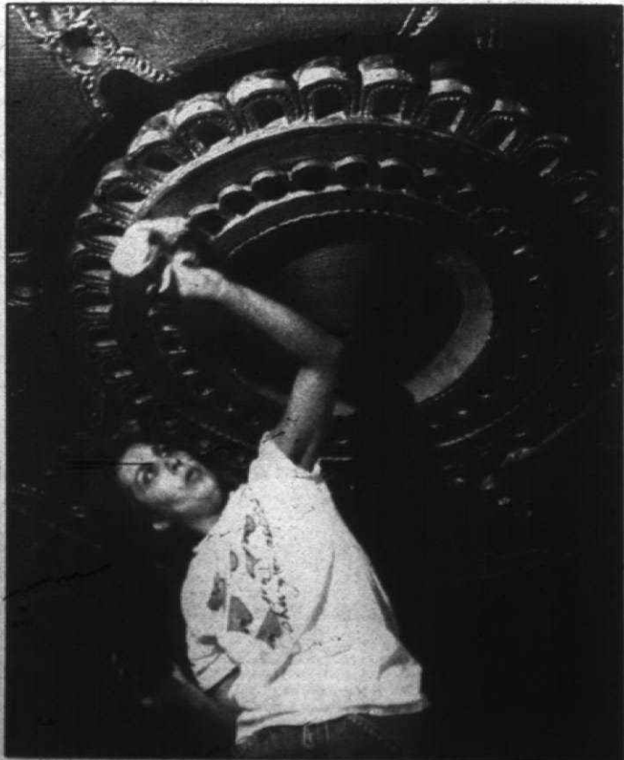
Sonya Winner applies linseed oil to the cleaned surface of the ceiling.
