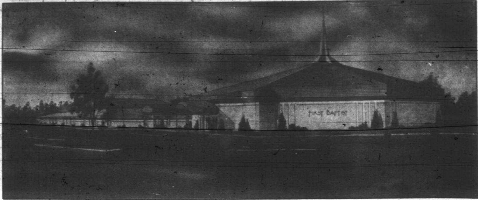
Cherry Hill and Sheldon soon will be home to First Baptist Church of Canton. The masonry and brick structure will face the corner, and there'll be 200 feet of landscaped frontage. Entrance will be from Sheldon Road and, eventually, from Cherry Hill as well.
