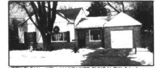
VERY CLEAN - WELL MAINTAINED BUNGALOW. 3 bedrooms, 1 1/2 baths, 1 1/2 car attached garage, double lot with fenced yard, newer furnace, close to shop and schools. $54,900 261-0700
