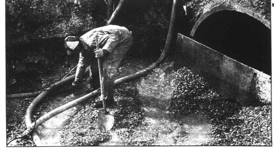
One would expect to find water in a drainage ditch but, in this case, the flow slowed down construction over the weekend on enclosing the Tonquish Creek. A worker is shown here Saturday pumping water.
