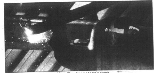
A construction worker arc-welds ceiling beams to framework.
