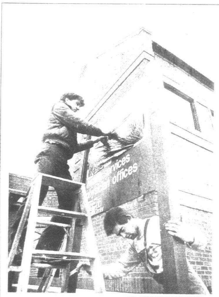
Ready to open Workers are putting on the finishing touches on the Huron Arbor medical health clinic under construction at Ann Arbor Trail and Harvey in Plymouth. Jim Masse of Livonia is shown here putting up a sign while Joe Gibbons of Plymouth tamps down the dirt holding the sign supports. The next day, Saturday, officials of Huron Arbor "wrapped" in ribbon to mark its opening.
