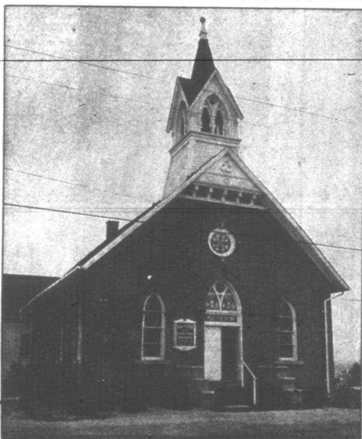
The old Cherry Hill United Methodist Church stands on Ridge Road in Canton Township.
