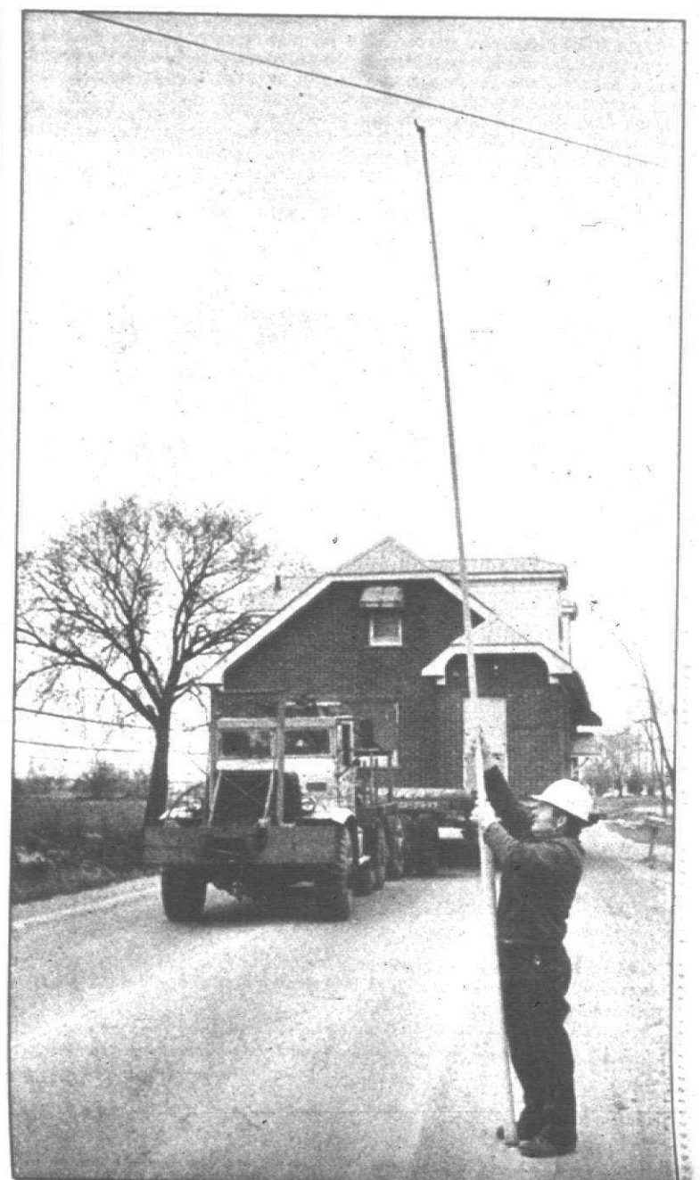
Utility workers lift wires out of the way or cut them to make room for the Christner house to pass underneath.
