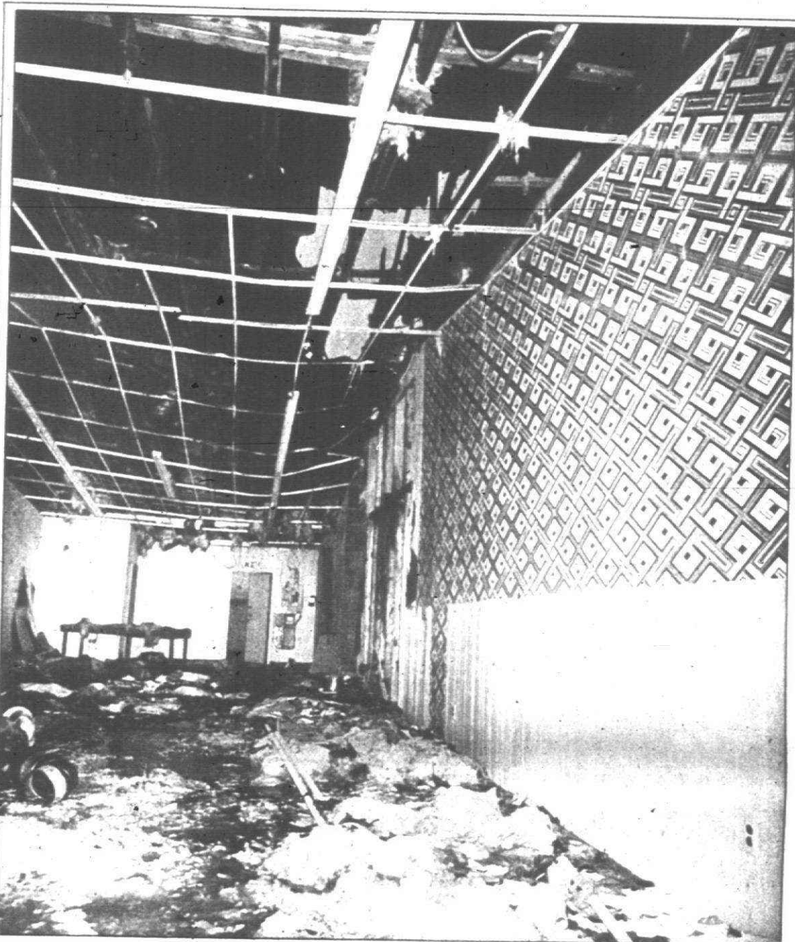
Water and ceiling materials lie scattered about the floor of one of the two stores damaged in a fire early Wednesday morning in the Kings Row Shopping Center in Canton. Fire officials estimated the blaze caused more than $65,000 in damage to the roof, walls and interior of C.W.'s Chicken and Ribs, where the fire apparently originated, and this adjacent vacant store.
