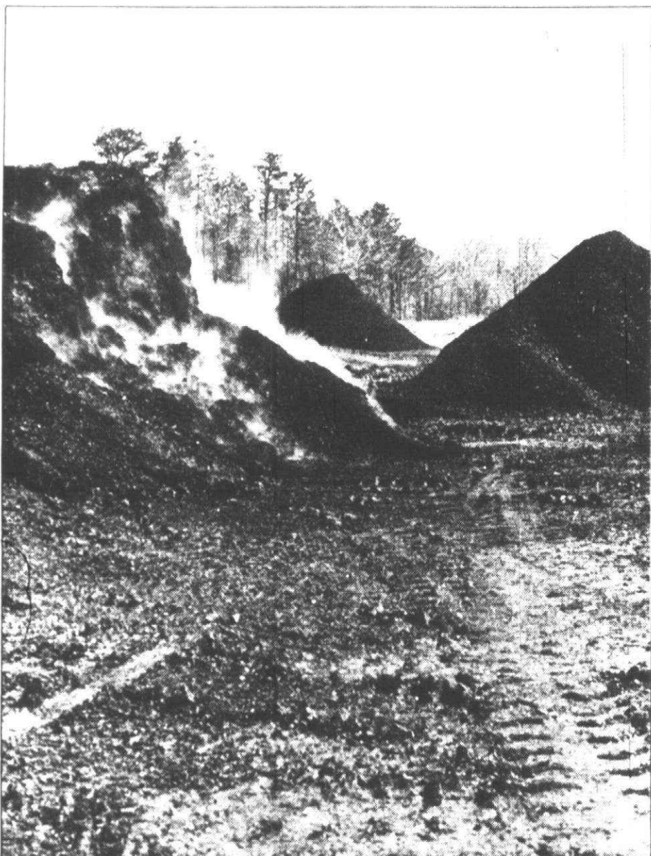
In the initial state, sludge is heat-treated (thus the steam) to destroy bacteria.
