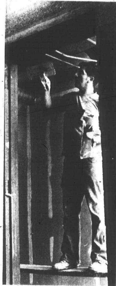
Putting the finishing touches on a door frame, this workman thinks twice while applying plaster.
