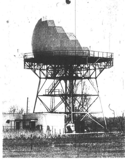
No one can enter the dome when the antennas are operating because of the high radiation. But over the past weekend, workmen entered the "golfball" to overhaul the moving parts that make up an important beacon for cross-country pilots. (Staff photos by Gary Caskey)
