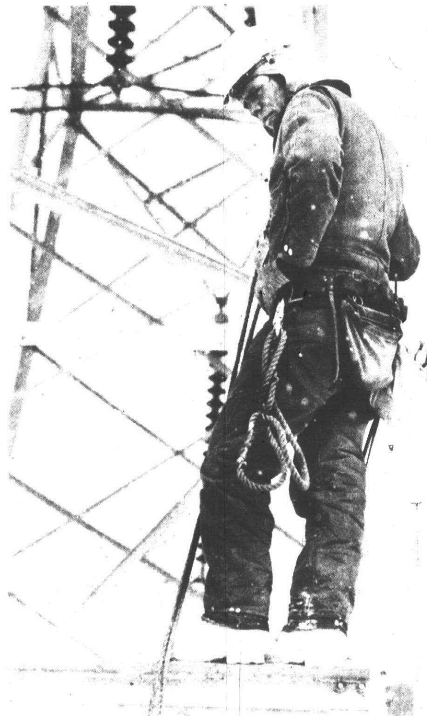
Edison worker Dave Patterson is stringing up high voltage lines that will whisk 345,000 volts of bulk electricity through the midsection of Canton Township. From the looks of things, he doesn't roll with the flow when someone calls him a live wire. (Staff photo by Gary Caskey)
