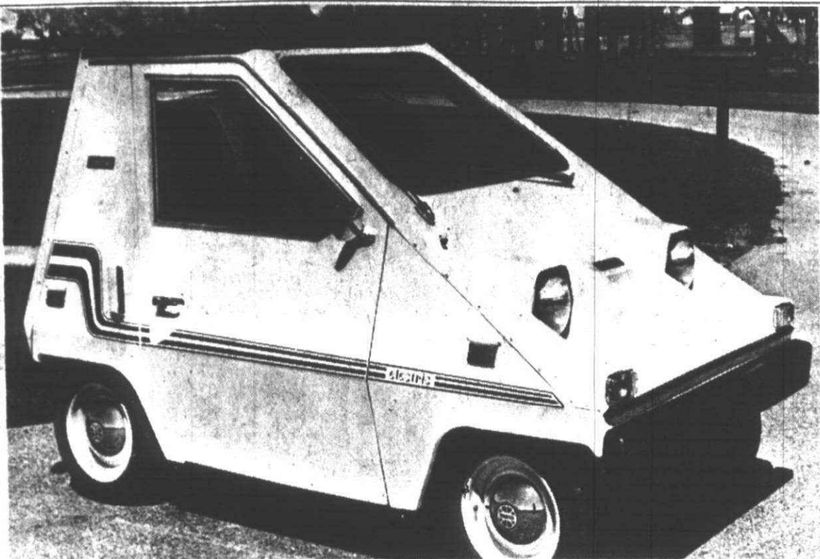
The CitiCar is coming—at under $3,000. The non-polluting electric car can go 40-50 miles on a charge, and has a top speed of 35 m.p.h.
