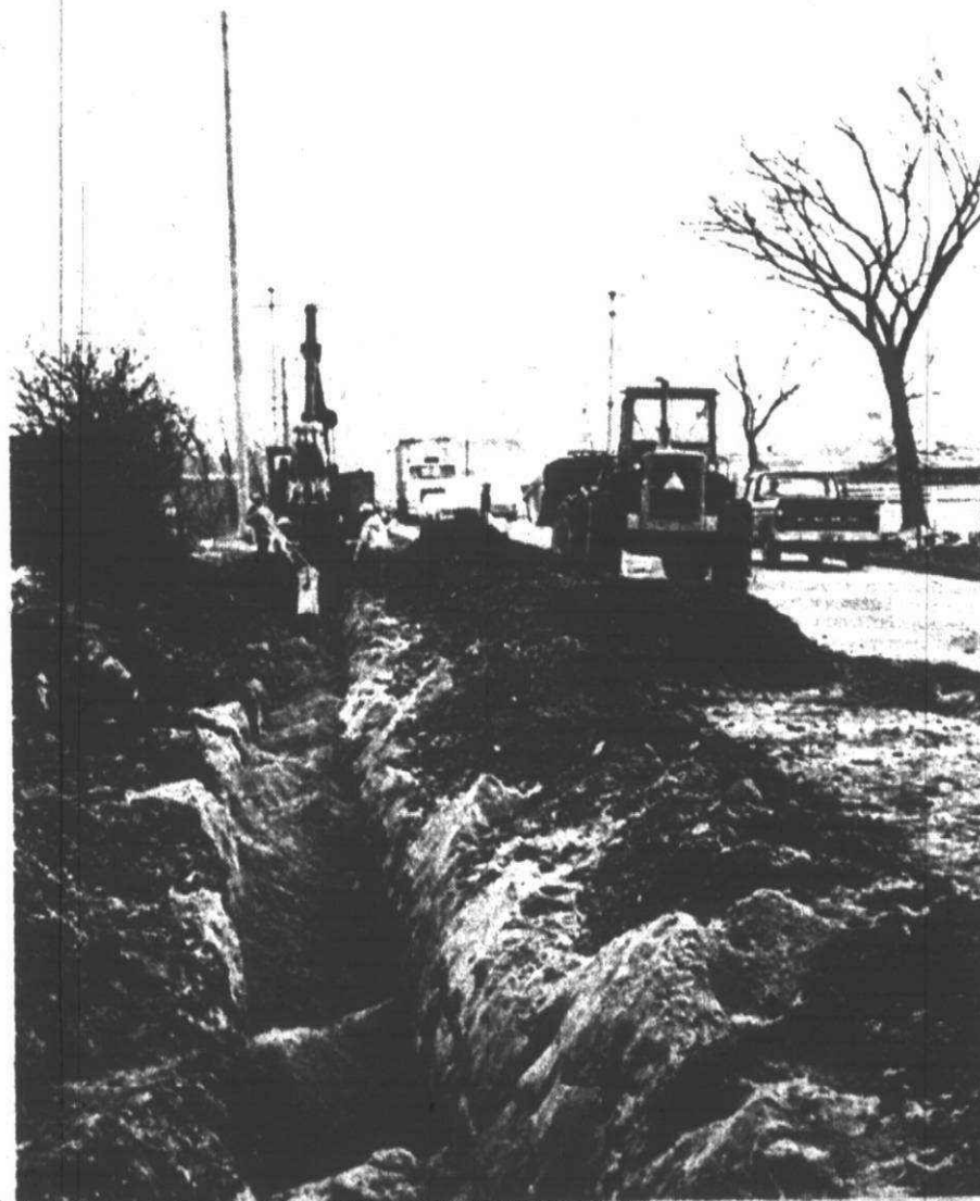
CONSTRUCTION OF a water main on Canton Center Road held up traffic this week, as workers laid the pipes that will connect the water systems in the southern and northern parts of the township. (Staff photo by Richard Gold.)
